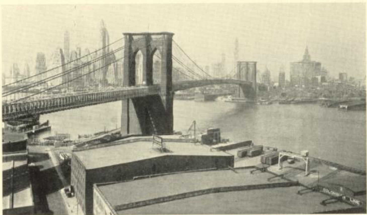
Brooklyn Bridge looking toward Manhattan—1933.
